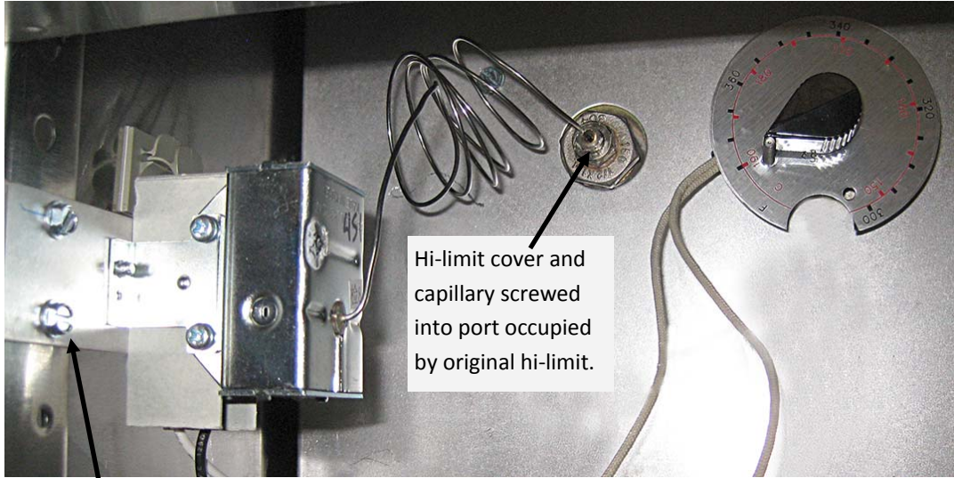
Hi-limit mounted in cabinet with drill-point screws.
